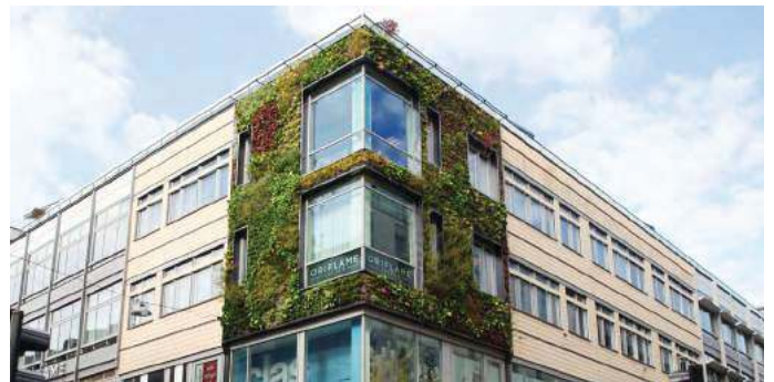
OUTDOOR PLANT WALLS
